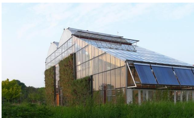
Figure 3. Increased height of greenhouse
